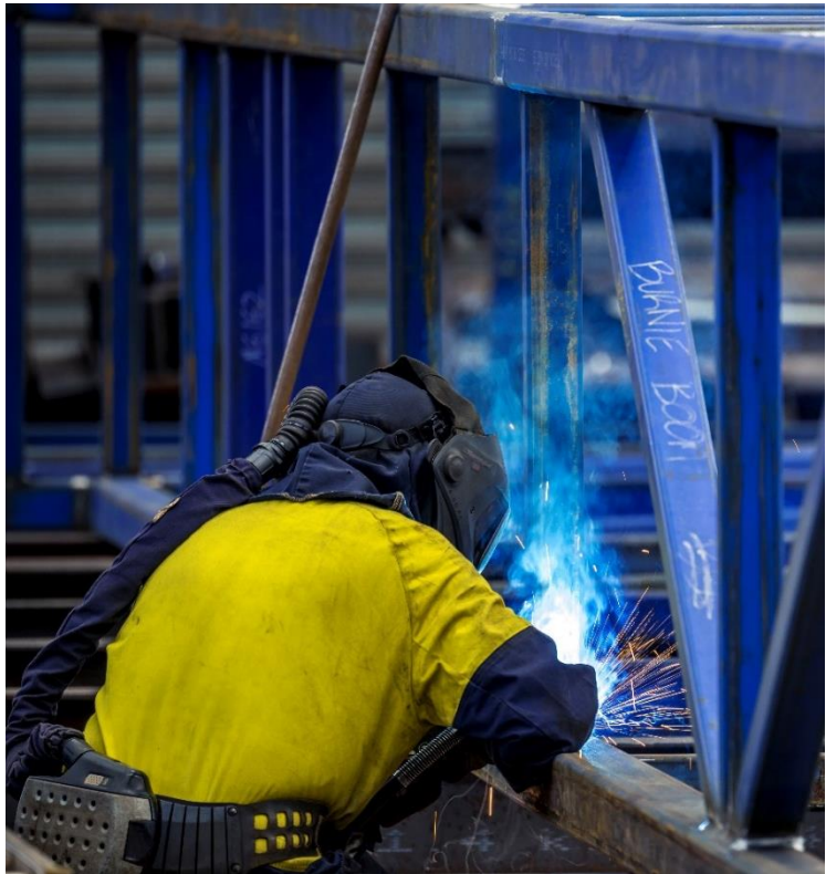
Figure 2: TasRail's shiploader project supports 140 design and construction jobs.
